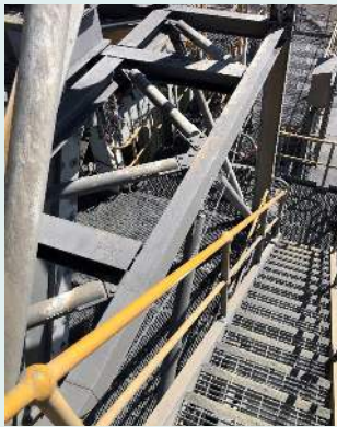
Walkway providing general access—AS 1657 applies
